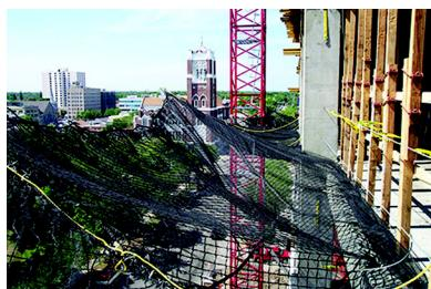
PearlWeave Personnel Safety Net Systems when installed horizontally provide passive fall protection for workers above the nets and passive Debris Netting protection for workers and the public below the nets.
