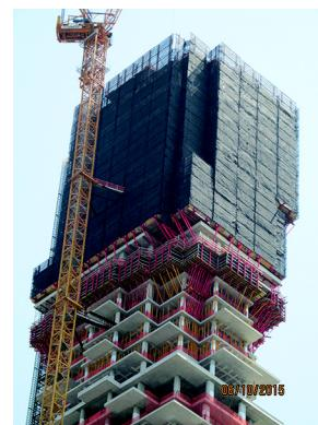
PearlWeave offers a full-line of OSHA compliant debris netting systems. Selection criteria for determining mesh construction and rated capacity are based on product weights/descriptions and fall distance/trajectory.
