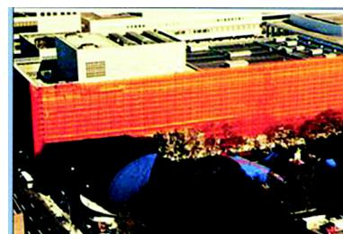
Designed to protect workers and pedestrians walking near the base of a scaffold structure. It also provides comfort for construction personnel by allowing air circulation. Scaffold netting allows most of the wind to pass through, so during windy conditions, it avoids excessive wind loads on the netting attachments or on the scaffold itself.
